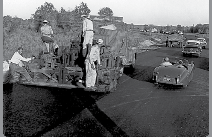
The widening of Highway 67 south of Malvern in 1956.
